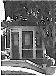
Ticket office for Te Runanga Tearooms. Converted to toilet in 1980s. No longer functional
