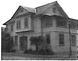
Wohlmann House – former Medical Superintendents House now part of RAVE complex
