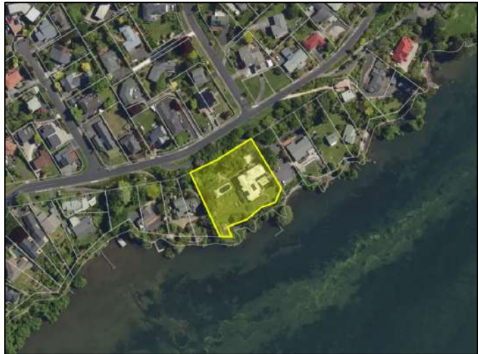
Figure 2 Black Swan Lakeside Boutique Hotel site
