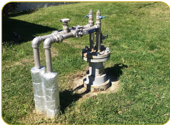
Figure 12 Bore examples. To the left is a typical heat exchange bore. In the example to the right the lower part of a gas vent can be seen at the top of the well (photos: Rotorua Well Drillers)
