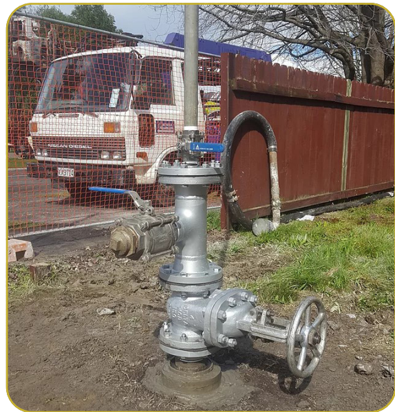
Figure 12 Bore examples. To the left is a typical heat exchange bore. In the example to the right the lower part of a gas vent can be seen at the top of the well (photos: Rotorua Well Drillers)
