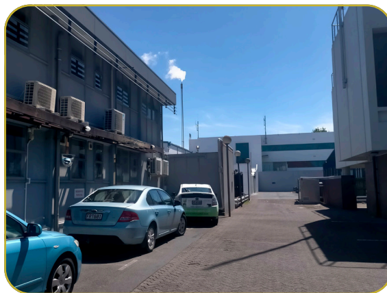
Figure 20 Geothermal venting structure (photo: Kim Smith, January 2024).
