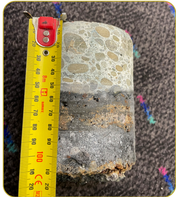
Figure 6 Concrete core showing effects of geothermal corrosion (Photo: Ash Bowtell)
