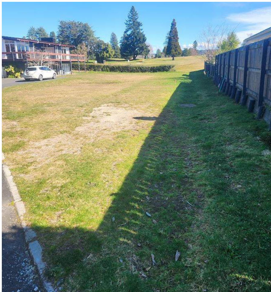
Figure 2. Grassed swale drain (shaded area) installed to consent conditions.
