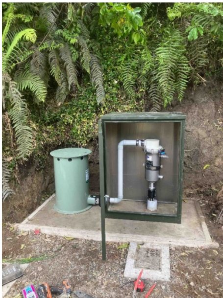
Air Valve Install Spencer Rd
