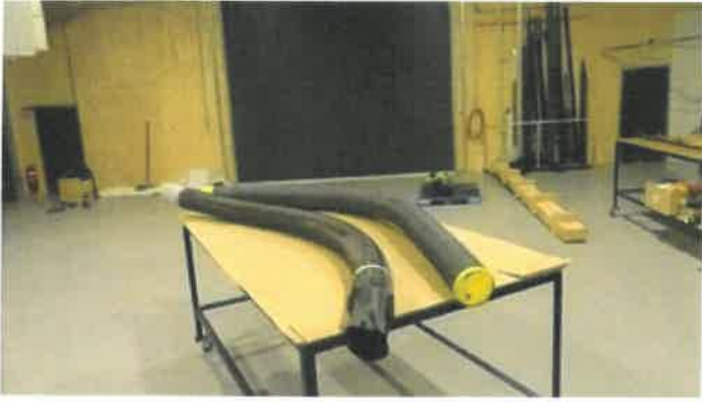
Above: the first couple of sections of the inner helix constructed
