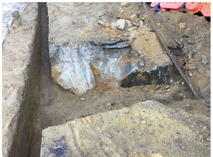
Rocks encountered during Saw cutting
