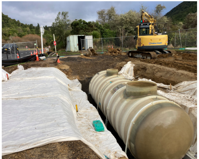
Transfer Station Pump Station – Holding tank installation
