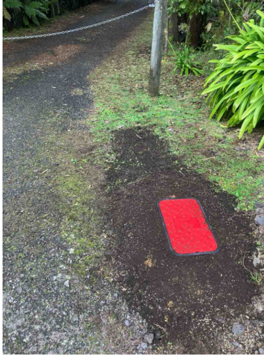
Boundary Assembly installation
