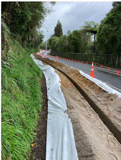
Saw cutting down Spencer Rd
