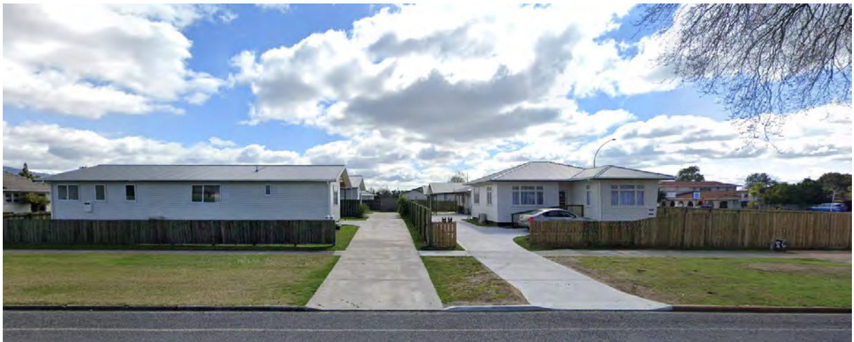
Figure 6: Image of 14, 16 & 16A Froude Street to the north of the subject site (Source: google Street View).
