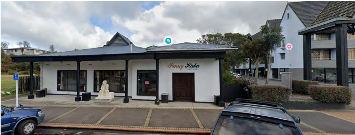
Figure 4: Image of the subject site (right) and the adjoining property to the south at 9 Tryon Street (Source: google Street View).
