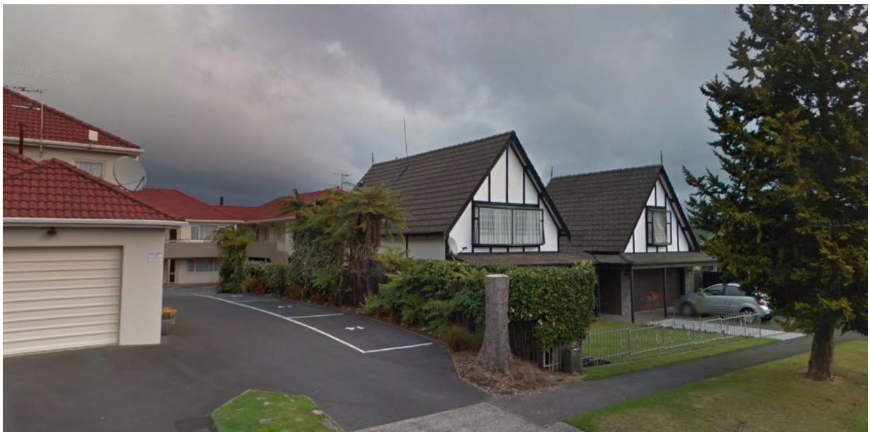
Figure 5: Image of the subject site (left) and the adjoining property to the west at 4 Robertson Street (Source: google Street View).
