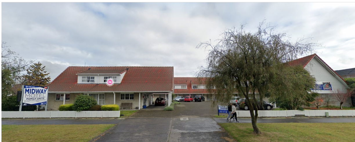
Figure 7: 293 Fenton Street streetscape from Fenton Street (source: Google Street View)
