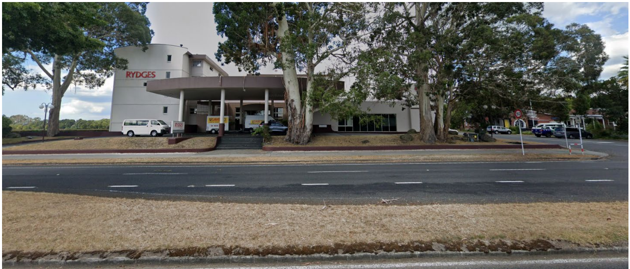
Figure 3: 272 Fenton Street – Rydges Hotel (source: Google Street View)
