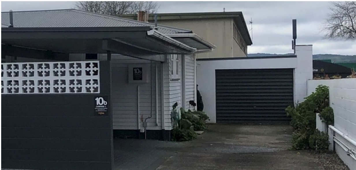
Figure 5: Driveway to 10C Toko Street showing the existing single garage at 10C Toko Street and parking area for 10B Toko Street.
