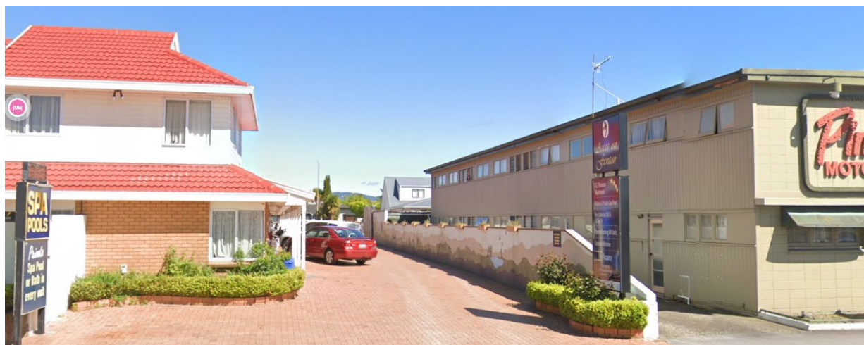
Figure 3: Streetscape view of subject site and adjacent property at 245 Fenton St
