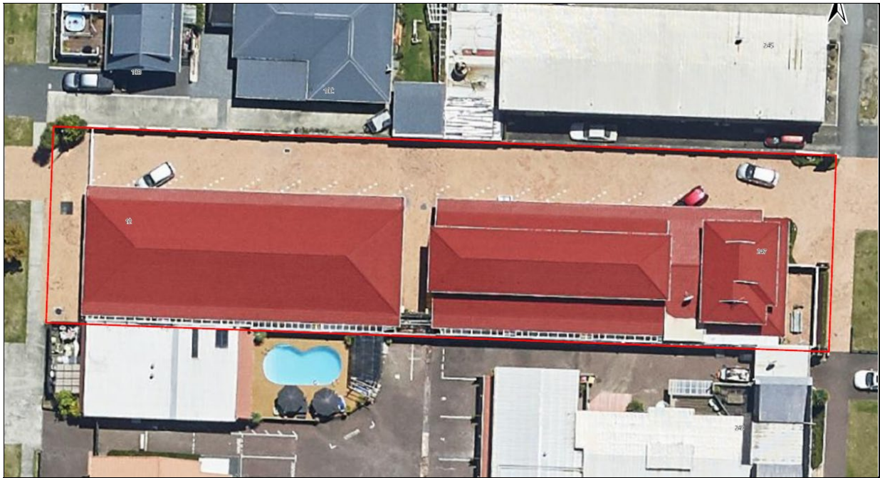
Figure 1: Aerial photograph of the site (Source: TPG Property Viewer)
