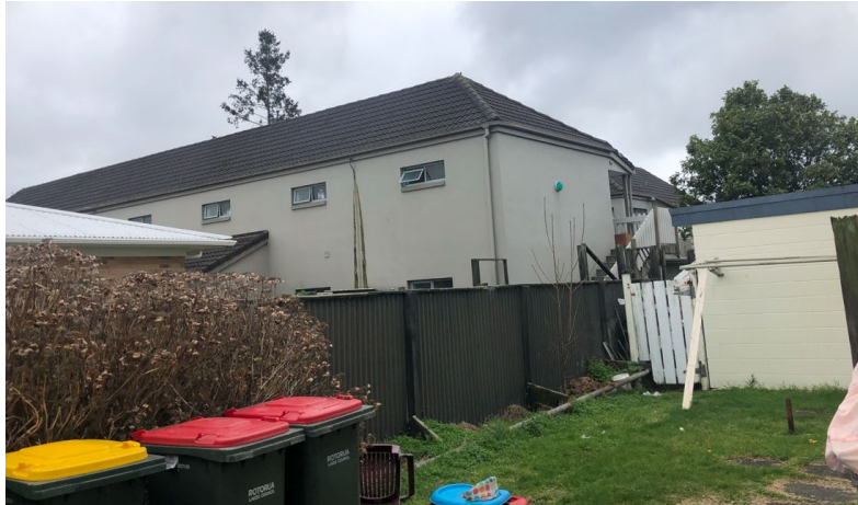
FIGURE 6: View from the subject site servicing area towards the Accolade Lodge at 30-32 Victoria Street
