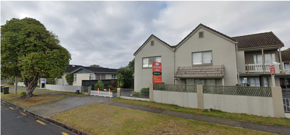
Figure 5: Image of the subject site (left) and the adjoining property to the west at 30-32 Victoria Street (Source: Google Street View)
