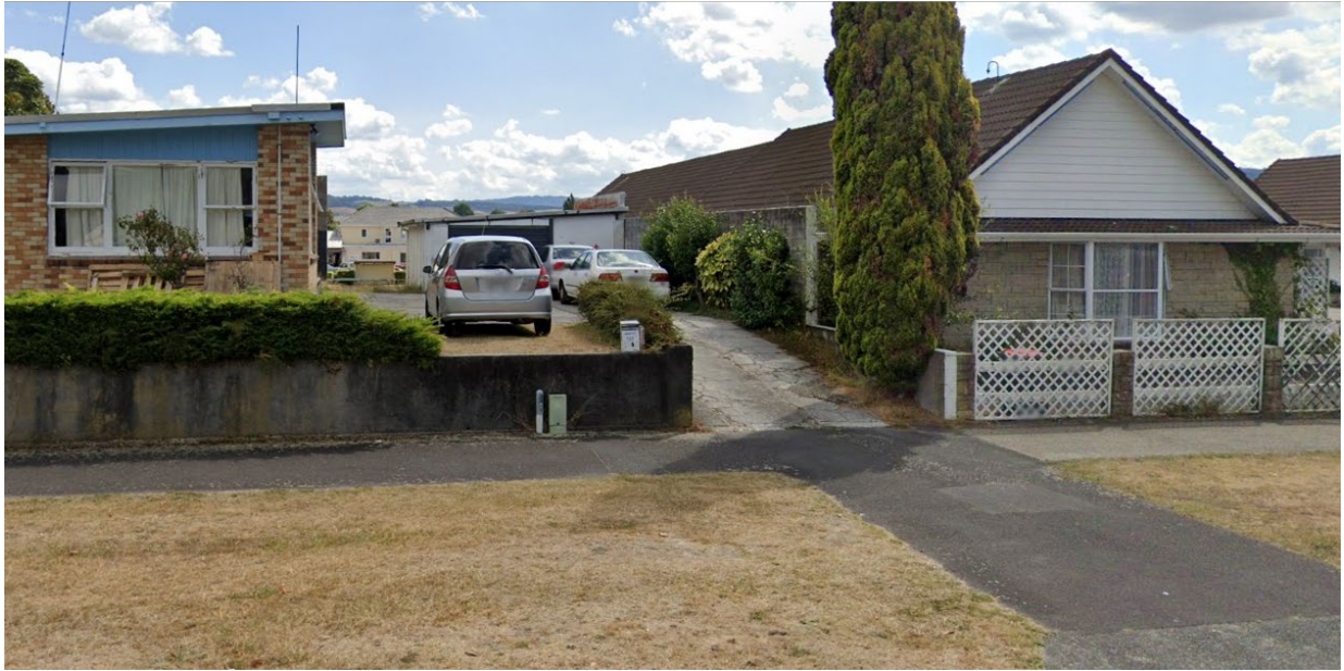
Figure 4: Image of the subject site (right) and the adjoining property to the south at 323 Fenton Street (Source: google Street View).
