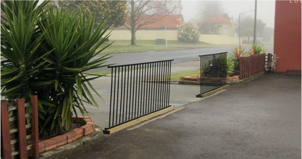
Figure 4: Security controlled gates at Ward Avenue frontage
