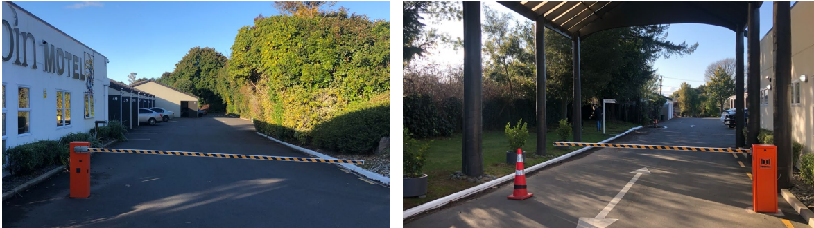
Figure 6: Barrier arm controlling vehicle entry / exit from the subject site
